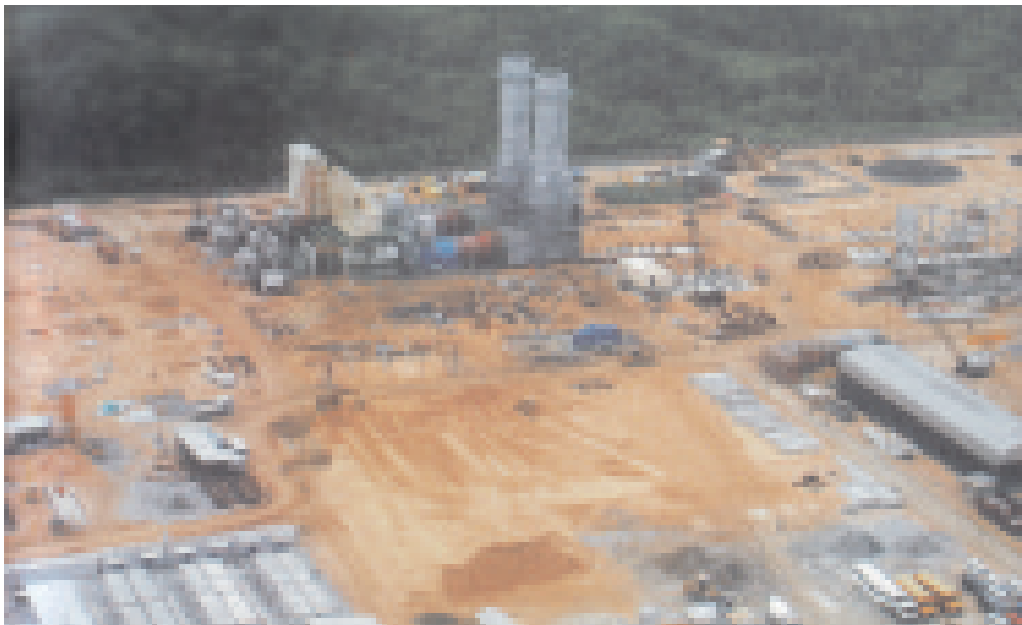
Okpai: Nigeria's power infrastructure is undergoing heavy construction
